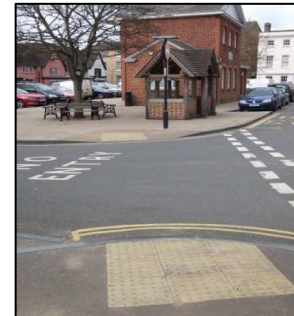
Dropped kerbs and tactile paving in Potton town centre
