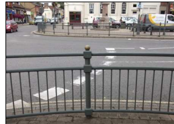
Guard railing on desire line in Biggleswade
